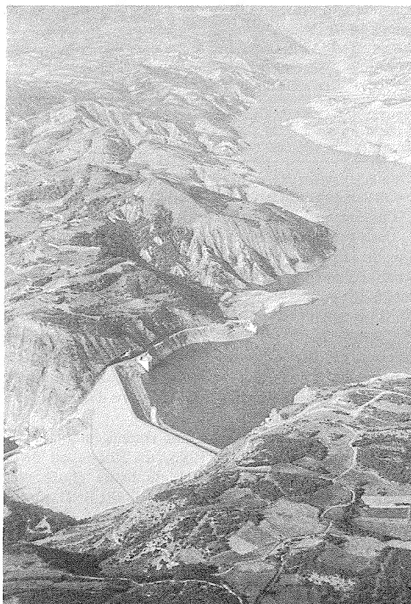
Figure 2 – Barrage de SERRE-PONCON (Durance).
