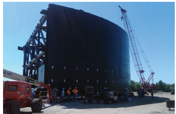
Figure 10: Sector Gate in Fabrication at Delcambre, LA.
