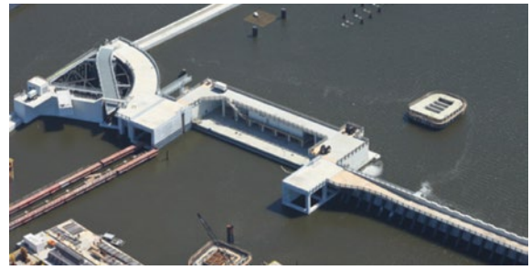
Figure 9: GIWW Bypass Barge Gate.
