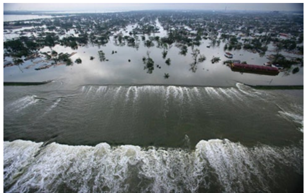
Figure 5: Hurricane Katrina Flood Wall Breach.
