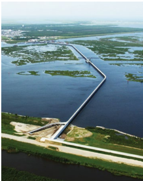
Figure 7: New Orleans' First Line of Defense: IHNC Lake Borgne Surge Barrier.
