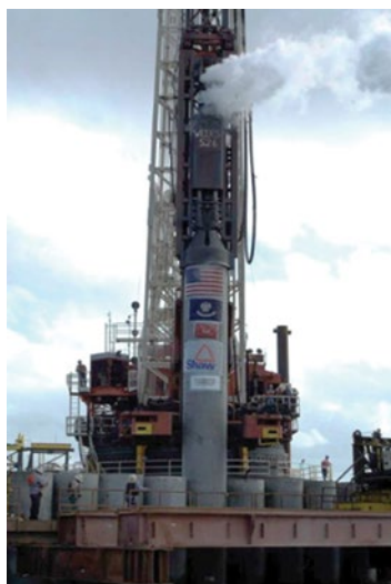
Figure 16: Final Pile Driven, October 23, 2009.
